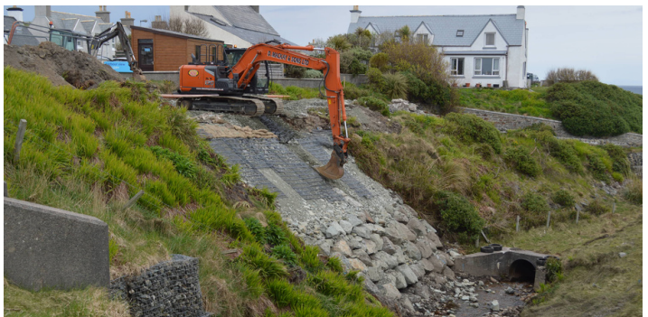
Reinstatement under way at Port of Ness
